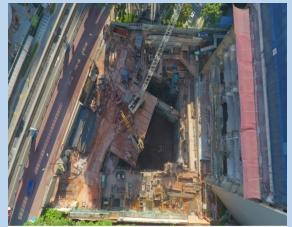
Probably one of the deepest underground basement ever constructed for a high-rise building in downtown Kuala Lumpur, a 37m-deep excavation was conducted for the upgrading of the MAS Building, on Jalan Sultan Ismail. The construction started with the demolition of the front podium of approximately 1,700m2 in area. The semi top-down construction method with kingposts was adopted akin to a strut-slab system, in place of the conventional steel strut and walers system.
